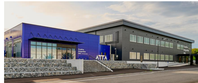
Exterior view of the Creative Integration Lab.™
